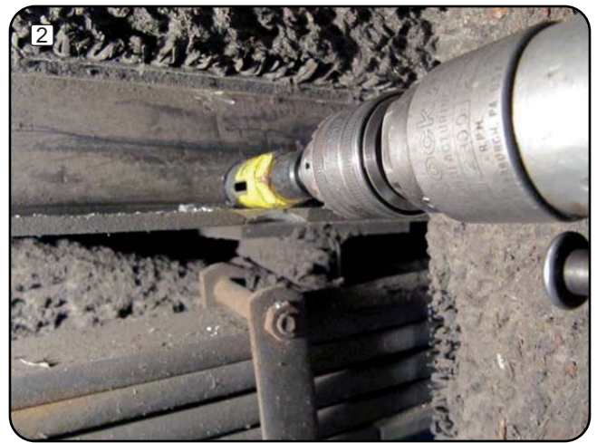
Drill 1" the web of the channel, as close as possible to the bottom flange.
