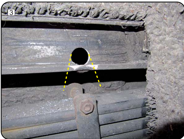
Using a reciprocating saw or equivalent tool, cut the flange flaring the bottom.
