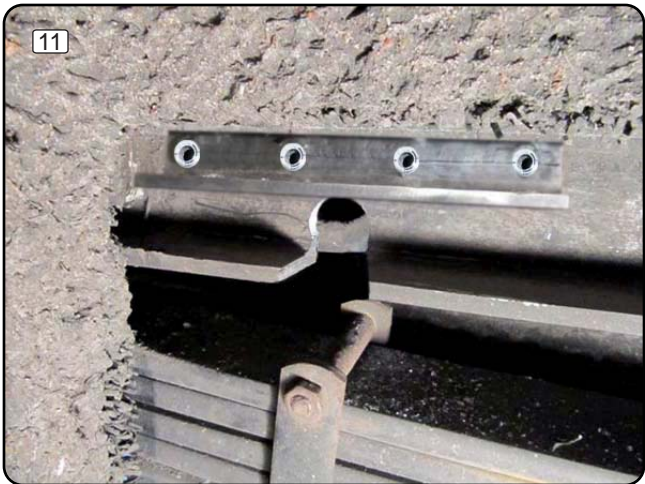
Place reinforcement provided with flange down, flush with the top of the opening, as shown.
