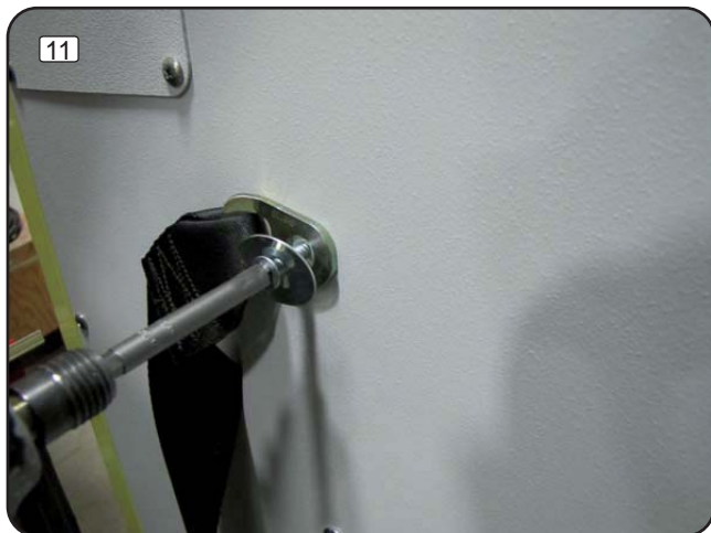
Reinstall the metal bracket with the same washer as shown.
