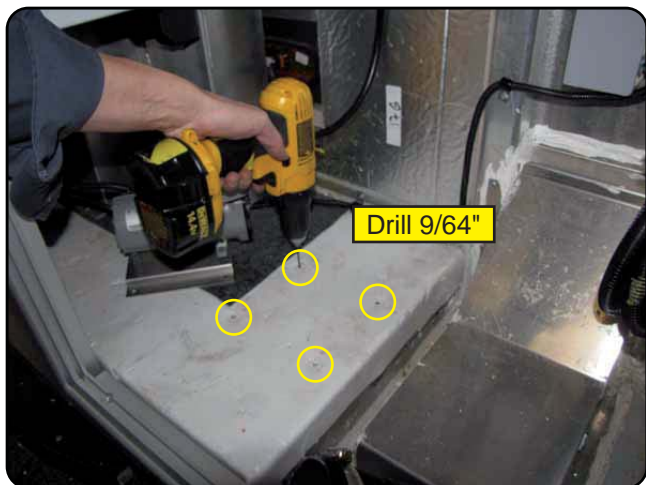
Drill 9/64" all the way through the metal.
