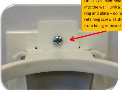
Drill a 1/8'' pilot hole through the mount ring and into the wall. Drill a 7/32'' hole through the mount ring and plate – do not drill into the wall. Install the retaining screw as shown. This will prevent the ring from being removed with the canister.
