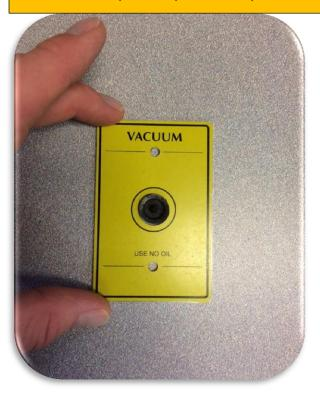
Use a hole saw to cut a 1 1/8" hole for vacuum hose. Drill appropriate size pilot holes for the retaining screws.
