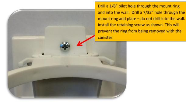
Install the new canister into the mounting ring.
