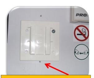
Install supplied wall mount plate – locate the plate just above the bottom hole where the previous suction unit mounted – use the wall mount plate as a template to drill the screw holes – install the supplied screws.
