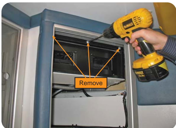
Remove the three (3) screws on the support.
